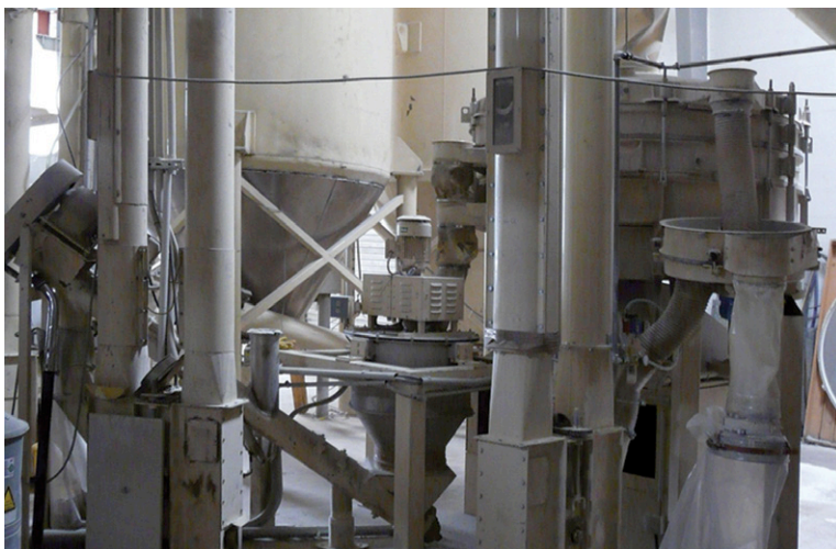
Below: As part of the Revinylfloor initiative, Aktion PVC-Recycling processed post-consumer flooring materials at its recycling plant in Troisdorf, Germany
